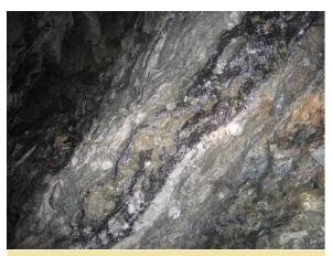
ABOVE: The gold ore at Charters Towers is visually very different to the host granite rock, and therefore relatively easy to follow for miners when excavating the tunnels in the ore in preparation for stoping (ore extraction).
